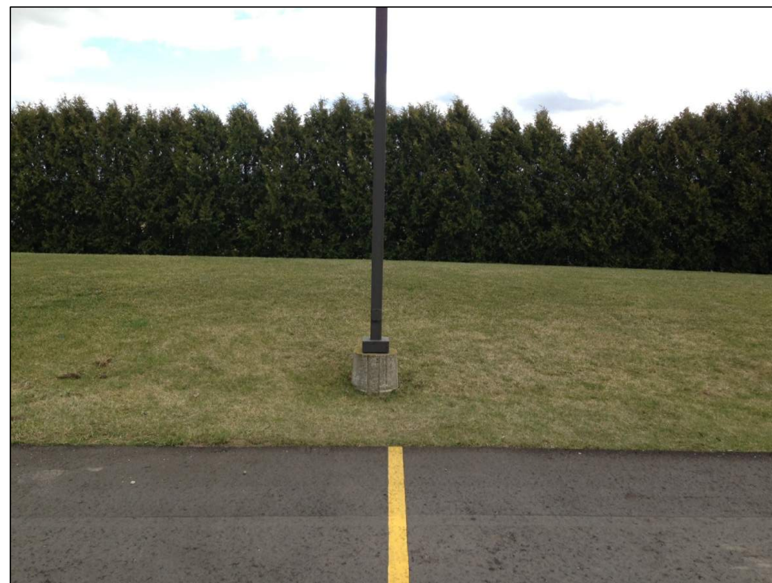
EXISTING LIGHT POLE BASE
