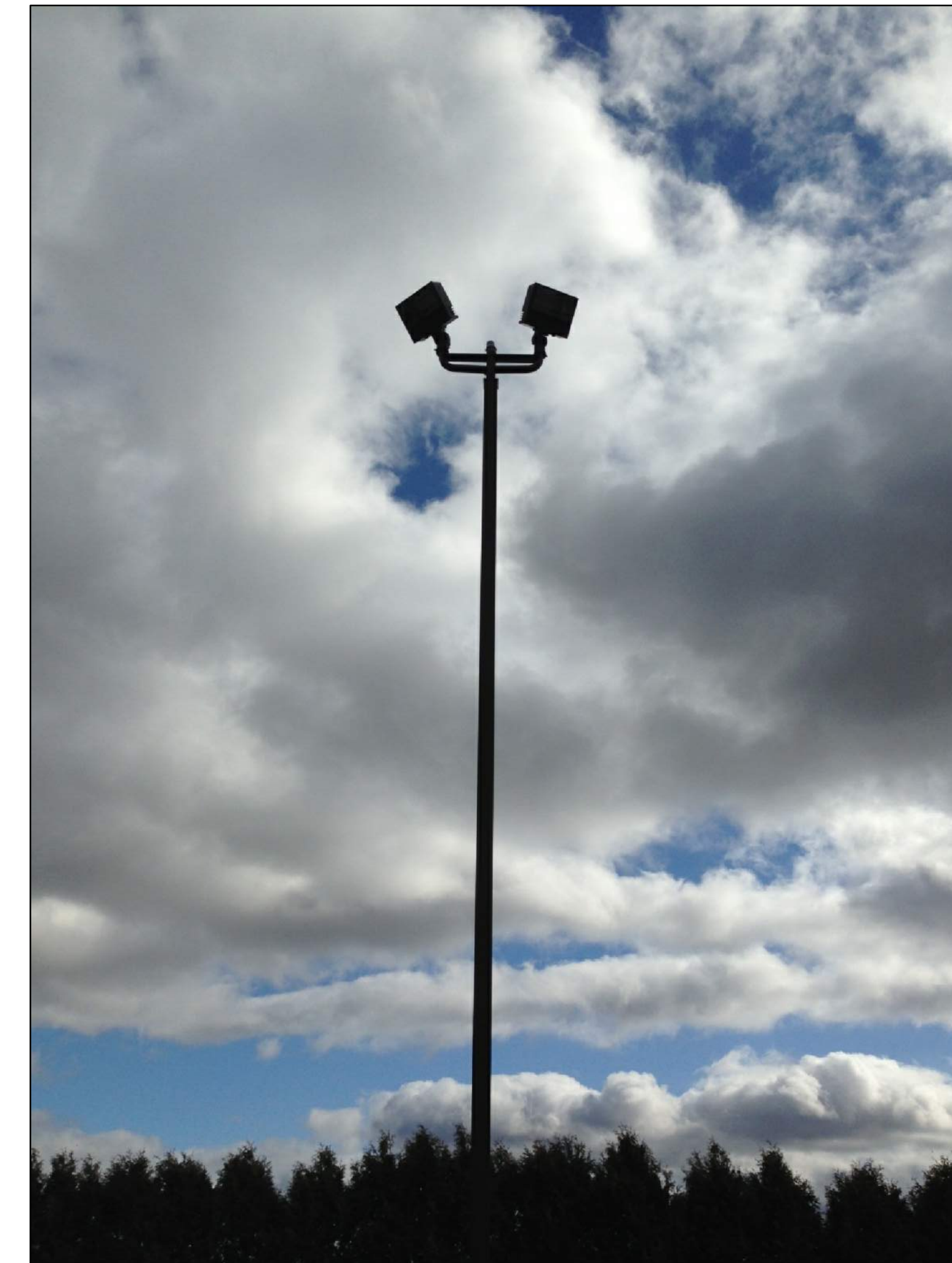
EXISTING LIGHT POLE FIXTURE
